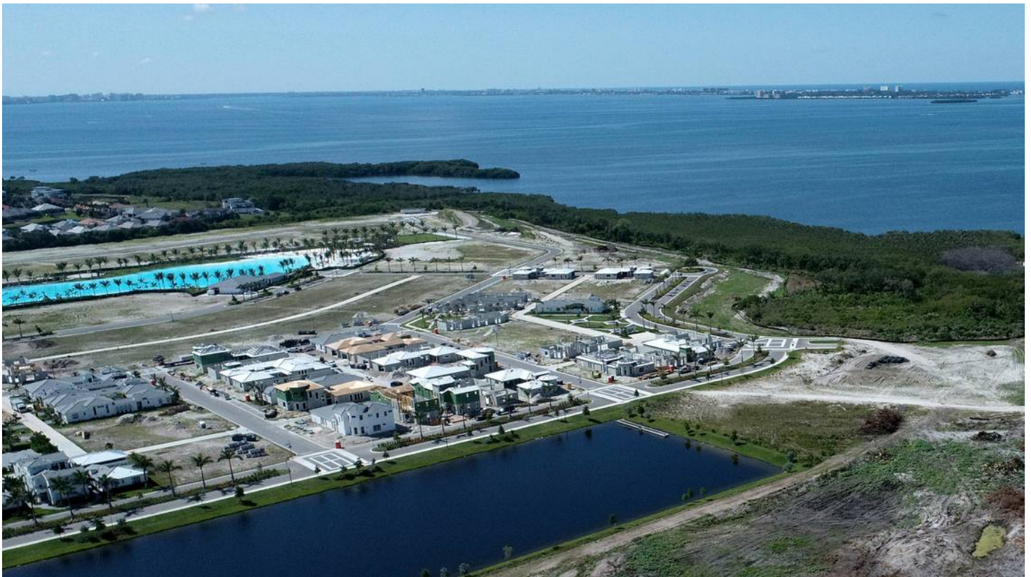
Local environmentalists have raised concerns over recent mangrove trimming along Sarasota Bay where Aqua by the Bay and Cirrus Apartments at Aqua are under construction on El Conquistador Blvd. Tiffany Tompkins ttompkins@bradenton.com
