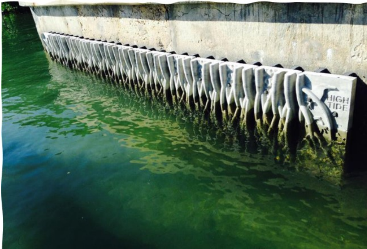
Example of mangrove panels on a seawall
