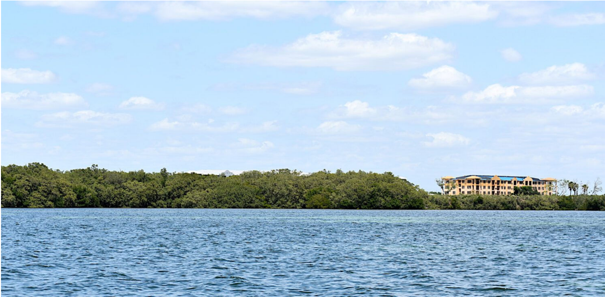
Some Aqua mangroves were trimmed to create better views for those occupying the development's multi-family residential buildings. – Joe Hendricks | Sun
