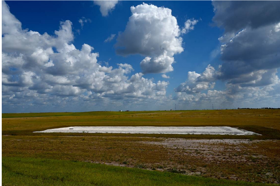
Site operators at Piney Point recently announced a milestone achievement with the closure of the Old Gypsum Stack-South compartment, one of four ponds that need to be closed at the former phosphate processing plant. The white area in the center is a drain to collect rainwater, while a complex seepage collection system is buried underground to collect and treat water trapped inside the stack. Tiffany Tompkins ttompkins@bradenton.com
