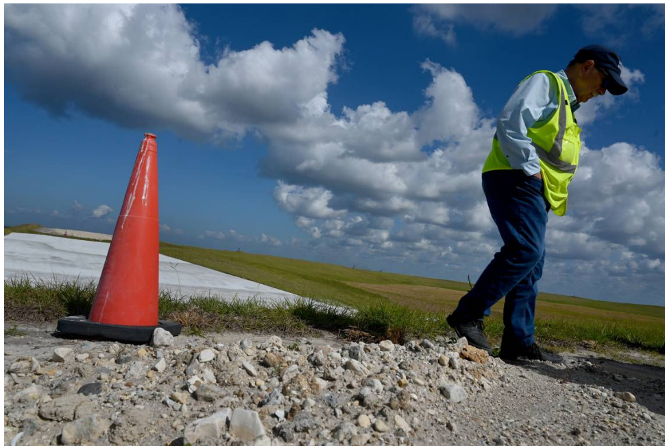
Site operators at Piney Point recently announced a milestone achievement with the closure of the Old Gypsum Stack-South compartment, one of four ponds that need to be closed at the former phosphate processing plant. The white pad to the left of Herb Donica is a weir, a ramp that prevents water from remaining in the pond. In the event of heavy rain, the pond is designed to overflow past the weir and into a stormwater collection area. Tiffany Tompkins ttompkins@bradenton.com
