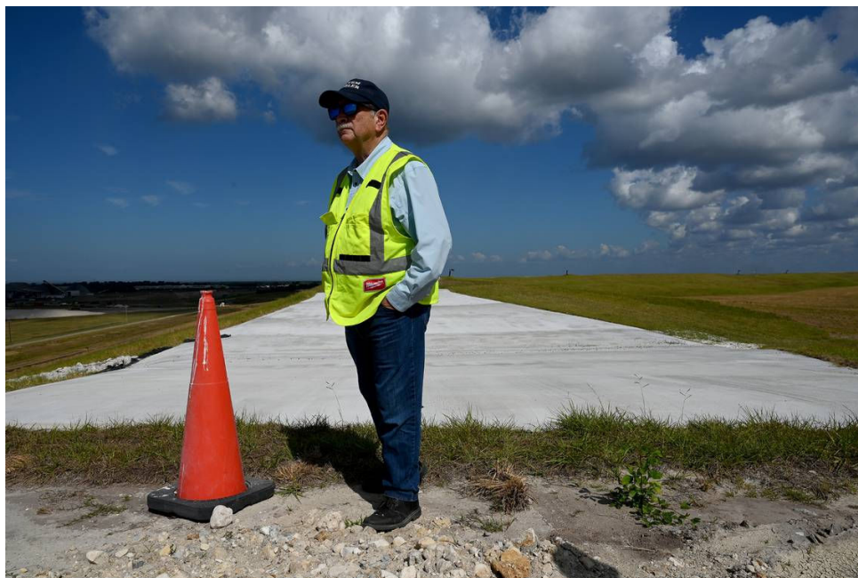
Site operators at Piney Point recently announced a milestone achievement with the closure of the Old Gypsum Stack-South compartment, one of four ponds that need to be closed at the former phosphate processing plant. The white pad to the left of Herb Donica is a weir, a ramp that prevents water from remaining in the pond. In the event of heavy rain, the pond is designed to overflow past the weir and into a stormwater collection area. Tiffany Tompkins ttompkins@bradenton.com
