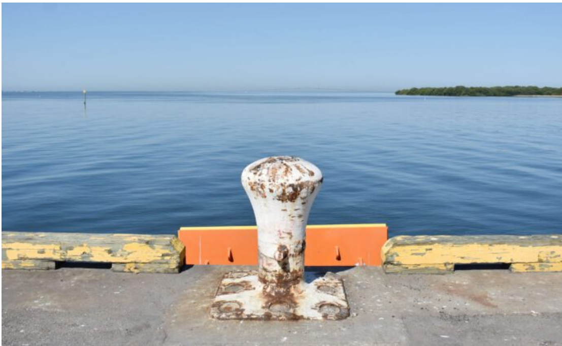
The salinity-infused Piney Point stormwater will be discharged into Tampa Bay at Port Manatee. – Joe Hendricks | Sun
