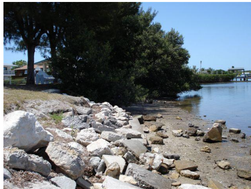
Original site with concrete rubble.
